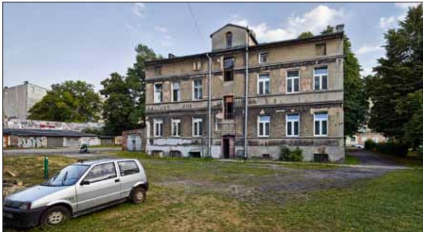
Former Fire Hall Field, Site of Speeches by Judenrat Head, Chaim Rumkowski, Zachodnia Street, Baluty, Lodz, 2013
